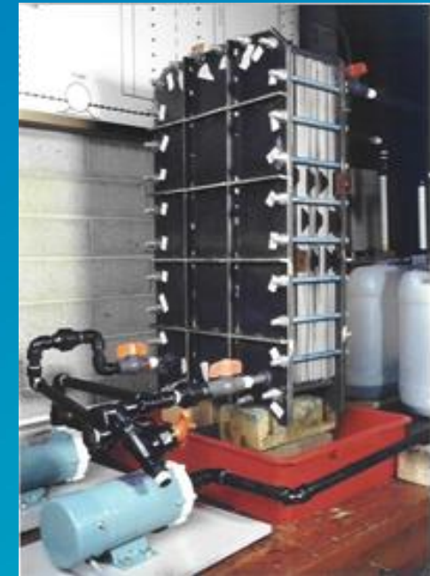
First 1 kW VFB multi-cell stack, 1988
